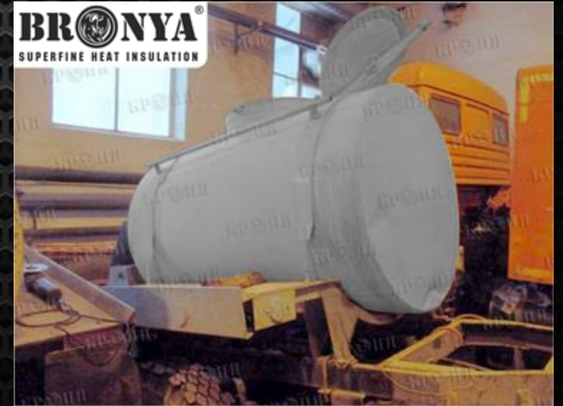
Permian. Insulation of a tanker
